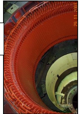
Core inspection; static components
